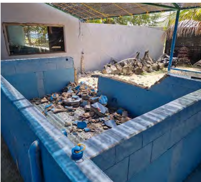
Above: Demolition of an older tank to make space for T5.
