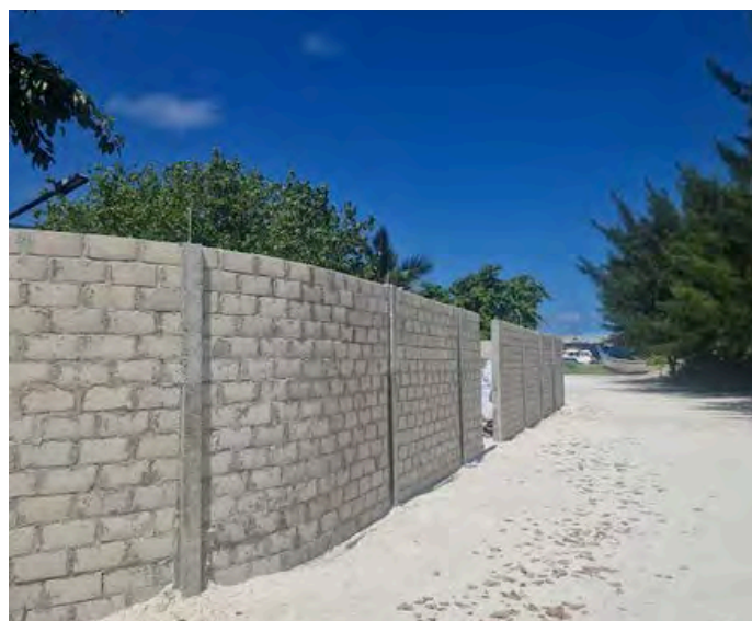
Above: AMC's outer wall under construction, July-August 2024.
