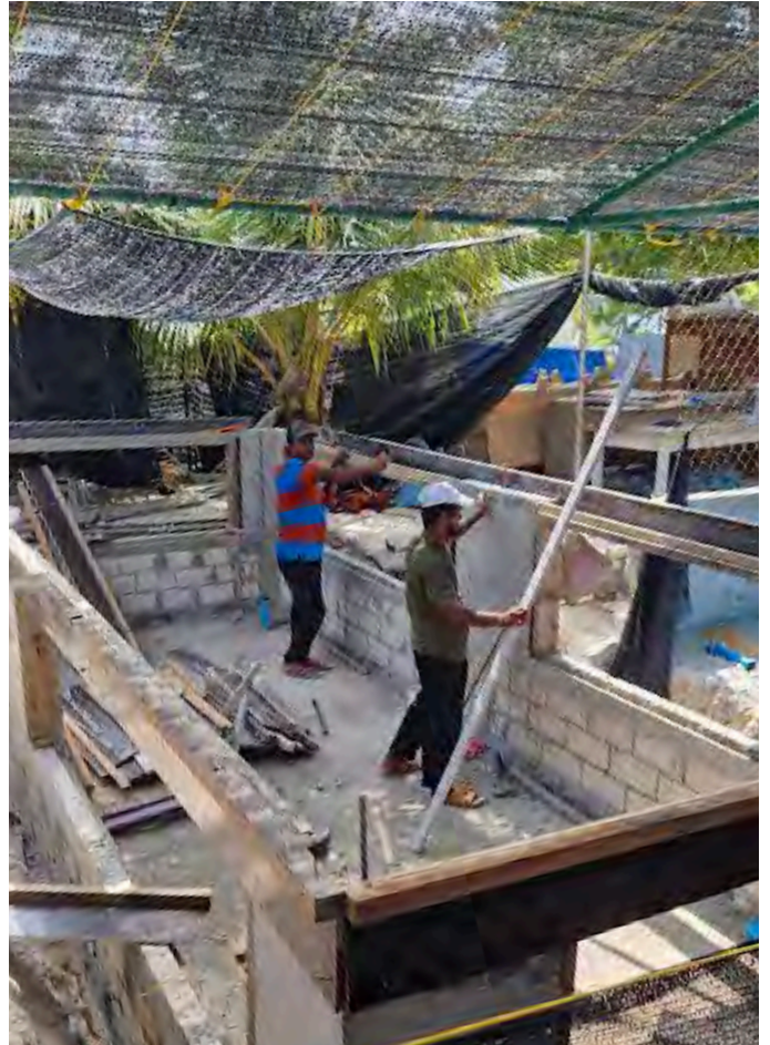
Above: Construction of T5 in progress during January 2024.
