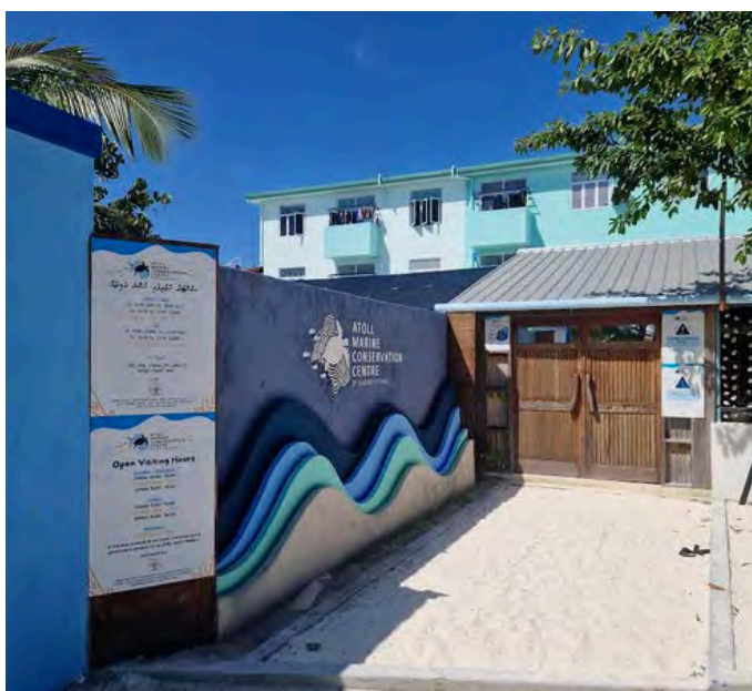
Above: AMC's outer wall complete, painted and sign-posted with opening hours, October 2024.
